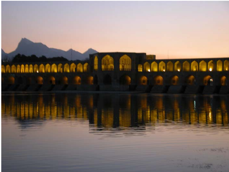
Bridge over the Zayandeh River, Esfahan
